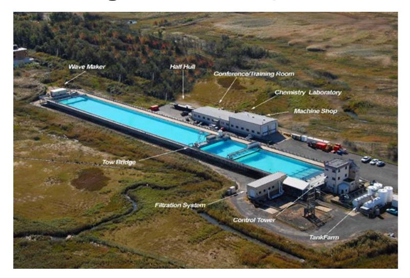
Ohmsett test tank: Length 200 m, width 20 m, depth 2.4 m and 9 500 m<sup>3</sup> of salt water. (5) SINTEF
