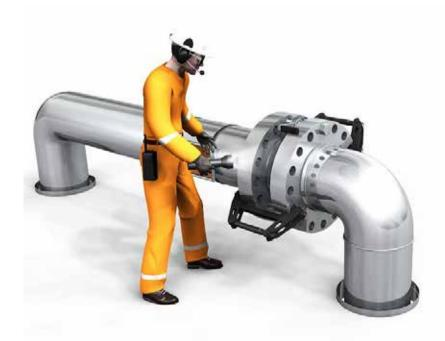
Immediately after the flanges are disassembled and cleaned, they should be inspected. Inspection personnel may need to be called in to perform a visual inspection of pipe/equipment and measure the ring track. If there is damage, this should be reported to a technical supervisor. Any tension in the pipe system should be reported to a technical supervisor.
