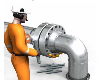
Metal rings (RTJ) shall be lubricated with a thin layer of acid-free Vaseline or thin machine oil before they are put in. This is so that point loads are avoided and so that it is easier to disassemble/remove the gasket again. Gaskets that are coated with PTFE should not be lubricated.
