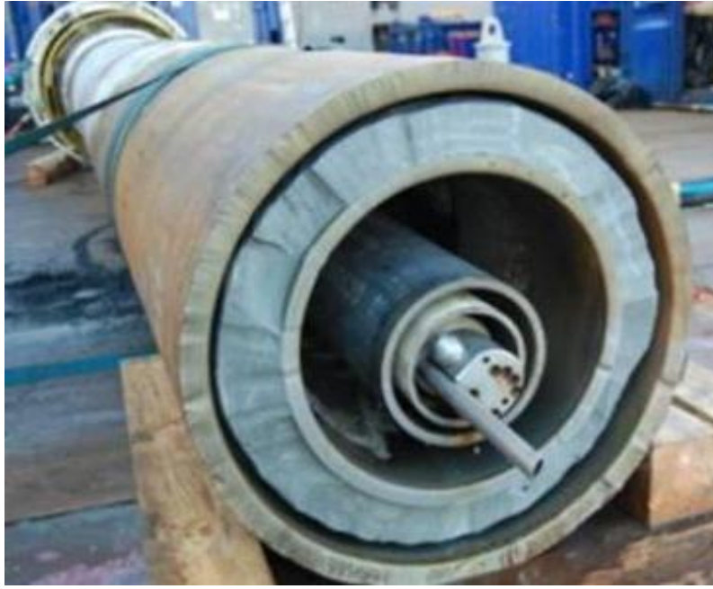
Figure 39: Picture of cut and retrieved intermediate casing, cemented production casing and tubing string with control line
