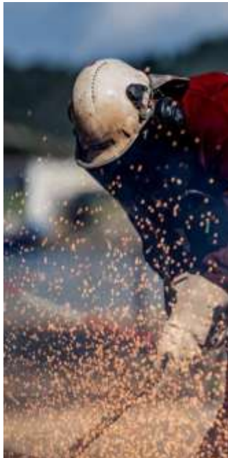
4. Removal, dismantling & segregation
