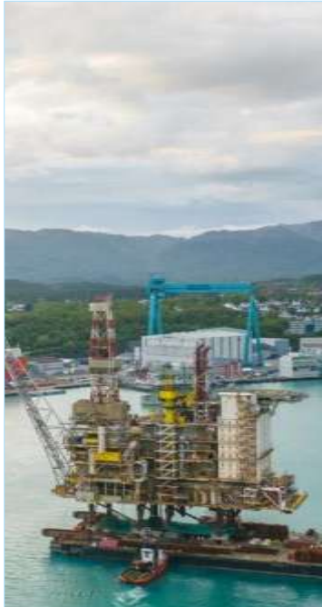
2. Receipt of structures
