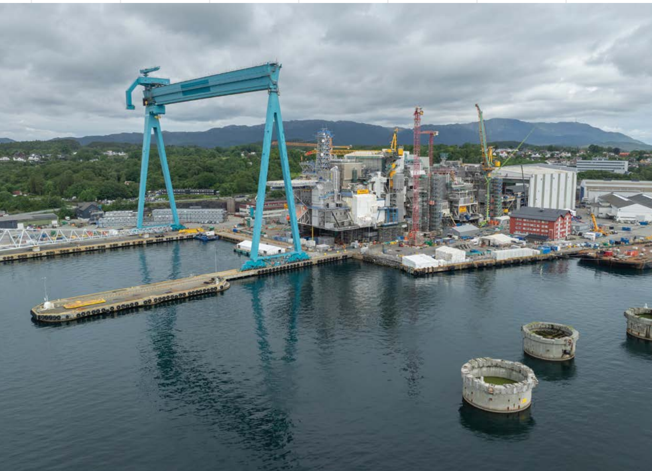
Construction of Hugin A and Valhall PWP on Stord. Photo: Aker Solutions
