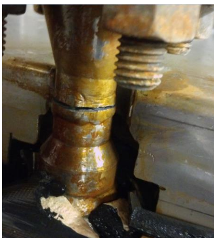
Figure 11 - Fracture in the weld on 1/2-inch pipe nozzle. Duplex steel.
