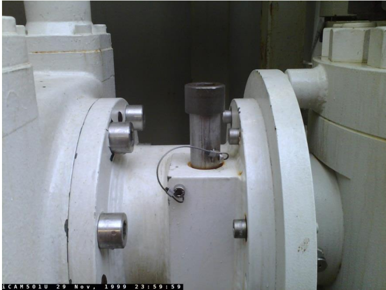
Figure 12 Example of a locking pin which physically locks a valve spindle. This prevents erroneous operation of the actuator changing the valve's position.
