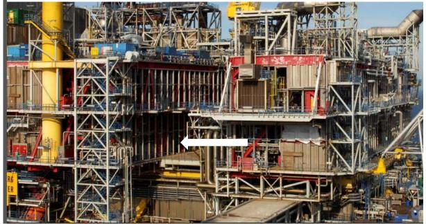
Figure 2 Process module M. The photograph is taken from Statoil's investigation report. The arrow has been superimposed to show where the leak occurred in M02.
