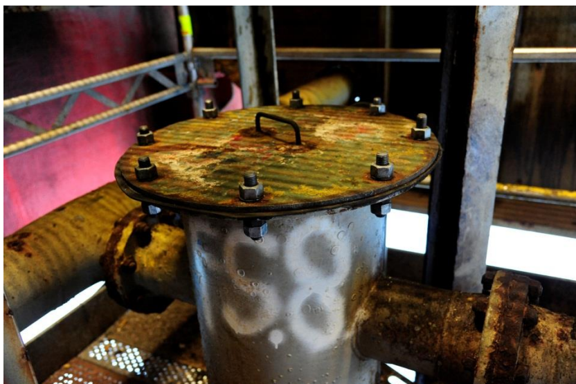
Figure 3. Photograph of fire seal FS8.
