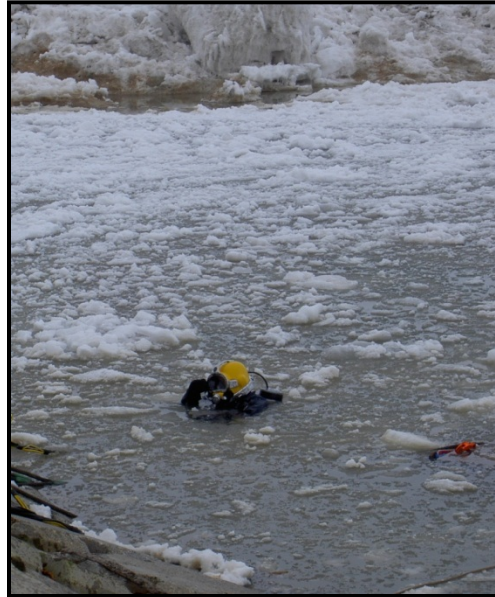
Conduct dive assessment to determine damage to blocks, filter fabric or geophysical barrier (gravel bags)
