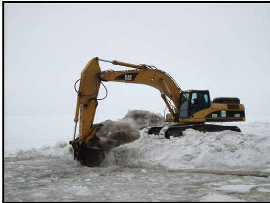
Excavate ice in work corridor
